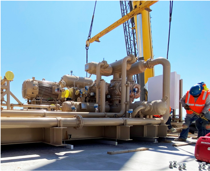
Field Service Base Installation
