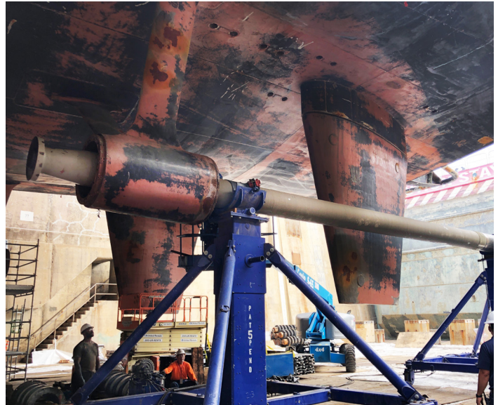
USS Rushmore (LSD47) - BENDER CCP provided propulsion system overhaul in San Diego and Vernon, CA
