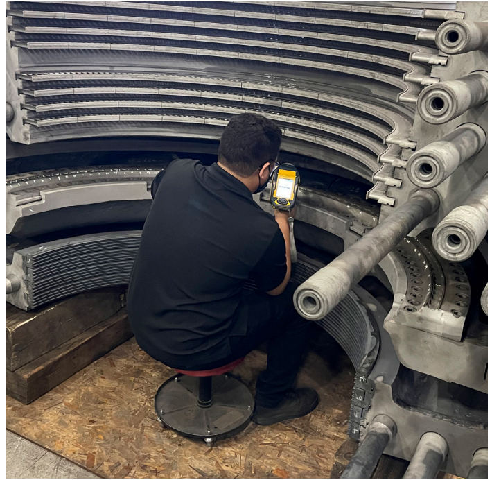
Performing PMI analysis prior to starting repair work
