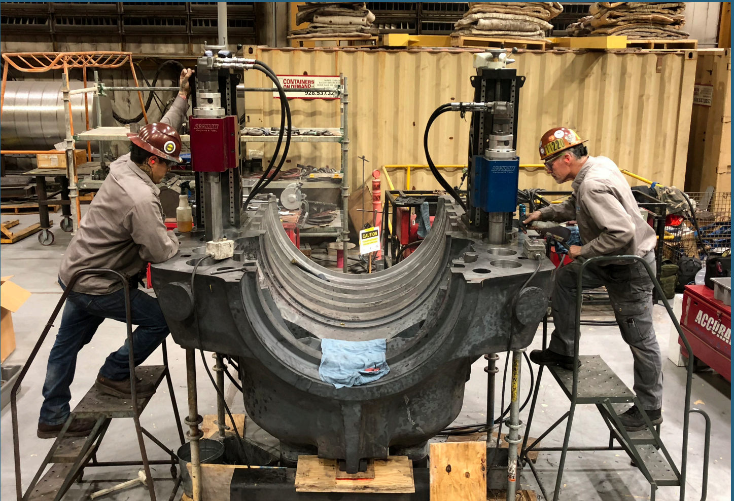
Removal of Studs Oversizing to an 8" Diameter
